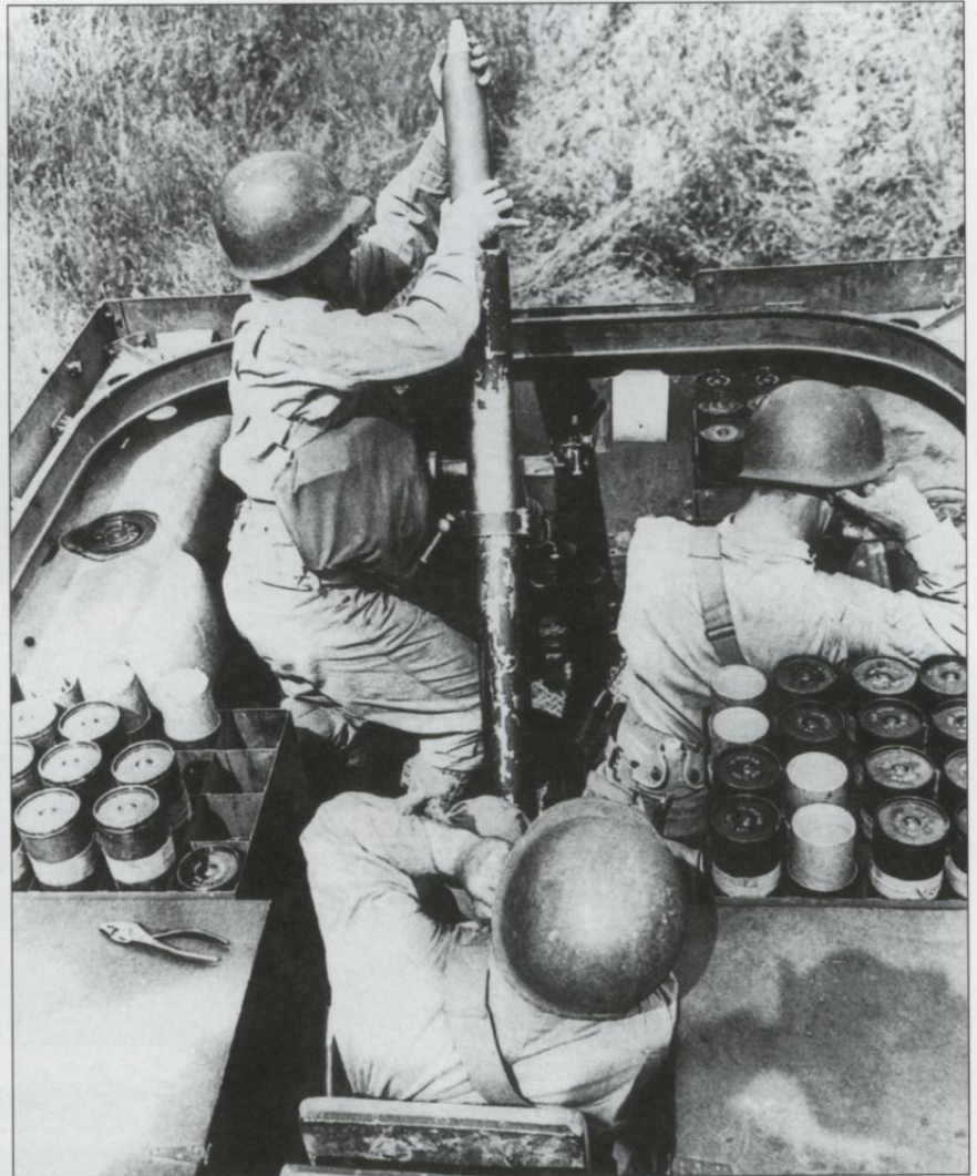
A M4 mortar motor carriage during stateside training. As is evident in this view, the mortar bombs came packed in fiber-board tubes. The mortar loader stood on the left of the mortar, the gunner to the right and the commander behind.
